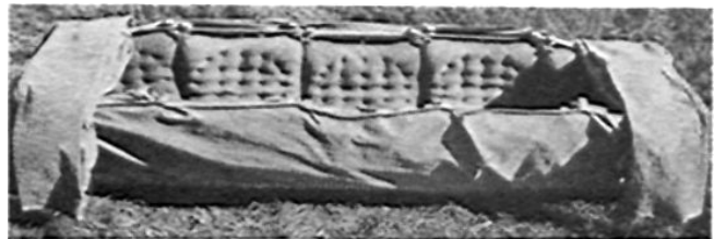
Figure 3. Canvas fitted snugly around saddles and tied to footrests.
